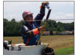
Install the Overhead AutoRANGER with a single hot stick.
