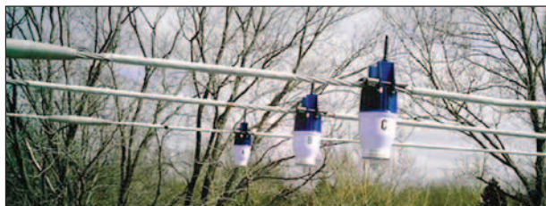
Wireless Sensor for Overhead Lines installation.
